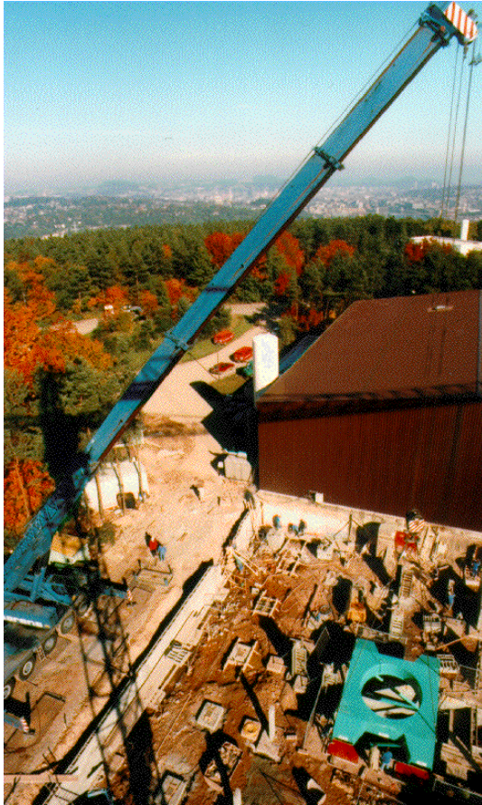
PICTURE 1 : Seismic block installation.
